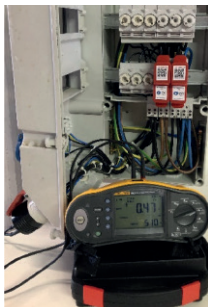
Loop impedance measurement on a subdistribution with CEE 16 adapter, measured with a test device according to DIN EN 61557-3 (VDE0413-3), (can be used independently of the manufacturer)
